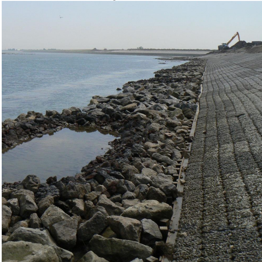
Figure 10 – Construction of the ecobasins (EcoShape, 2024e).
