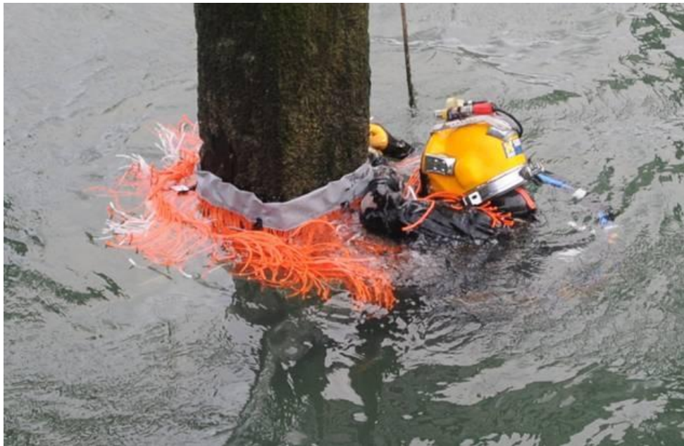
Figure 5 – Installation of polehulas (EcoShape, 2024d).
