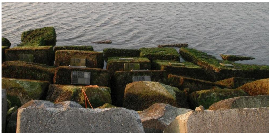
Figure 9 – Eco-concrete breakwater structures (EcoShape, 2024c).
