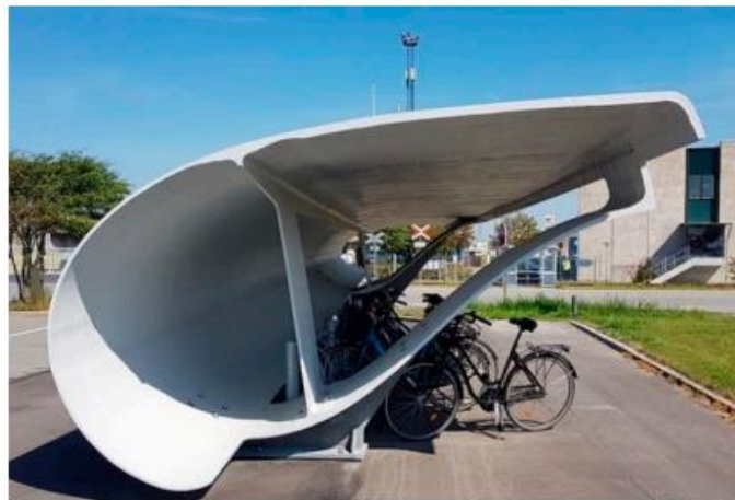
Figure 3 - A bike shed in Denmark made from wind turbine blades [26].
