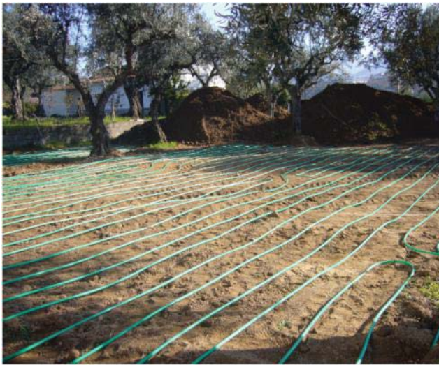
Figure 9. Horizontal geothermal capture.
