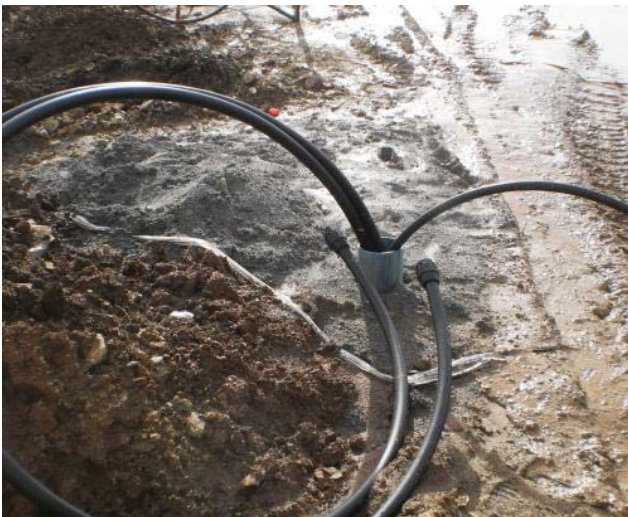
Figure 10. Vertical geothermal capture.
