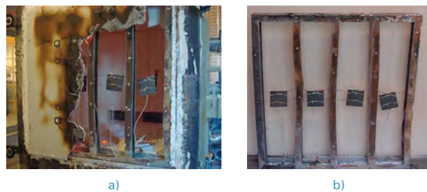
Figure 4. Final state of the wall and the steel structure (after 60 minutes of fire exposure).
