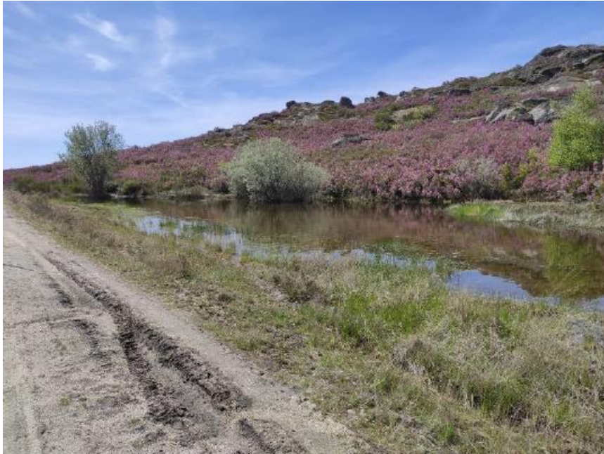
Figure 22. Accumulated water next to the unpaved Montesinho EBVT in 2023 (Kolodi 2023)
