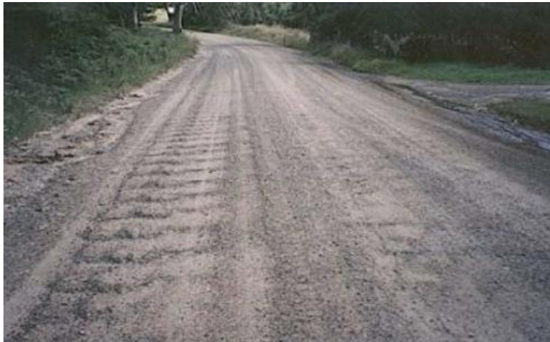
Figure 16. Photograph of an unpaved road with a corrugated surface (Andrews, Mathias, et Austroads 2009)
