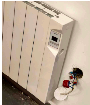
Fig. 4: Actuator installation.
