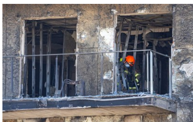
Figure 1: Fire in a LSF building in Valencia (Spain) (photo from El Pais, Mònica Torres).
