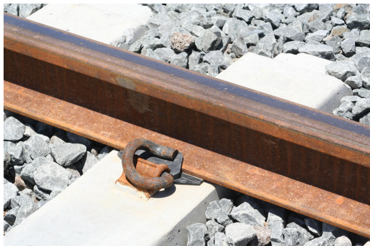
Figure 2.9 – Elastic Pandrol fastening.
