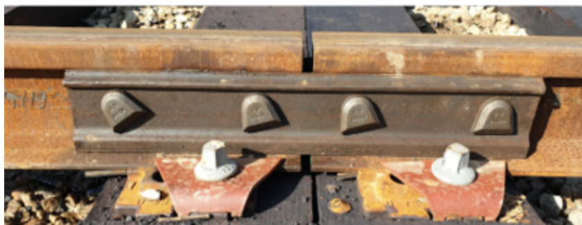
Figure 2.10 – Fishplate joint.
