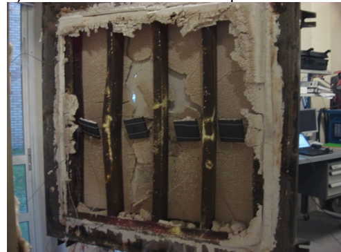
d) Final state of the LSF wall specimen 02.
