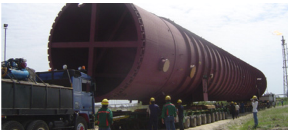
Figure 1.7. Deisohexanizer column: height = 57 m, diameter = 7 m, weight = 221 tons. (ESSAR Oil, www.essar.com )
