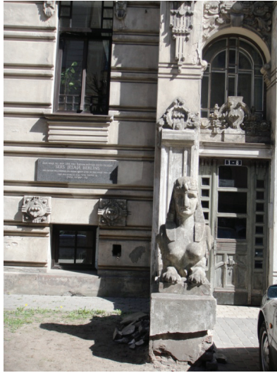
Figure 2 – Entrance to Berlin's house building 2A
