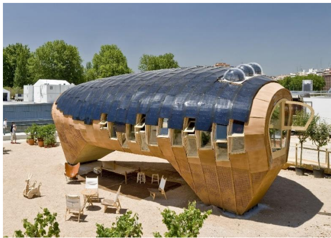
Figura 2 - Fab Lab House Barcelona (8)
