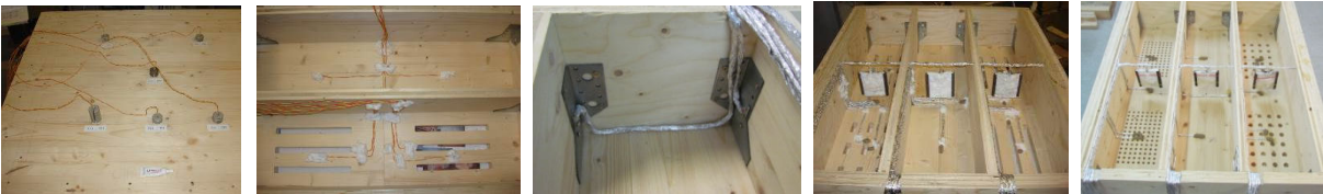
Fig. 5 - Thermocouples installation in wooden slabs.
