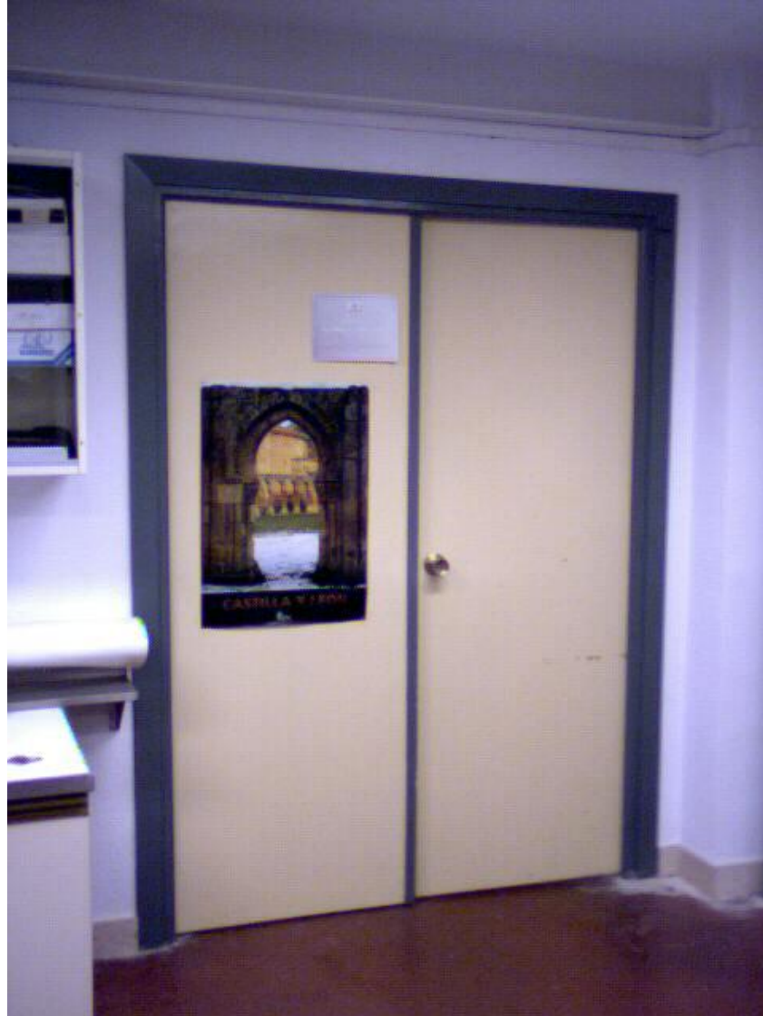
Figure 6.14 View of the tested door.
