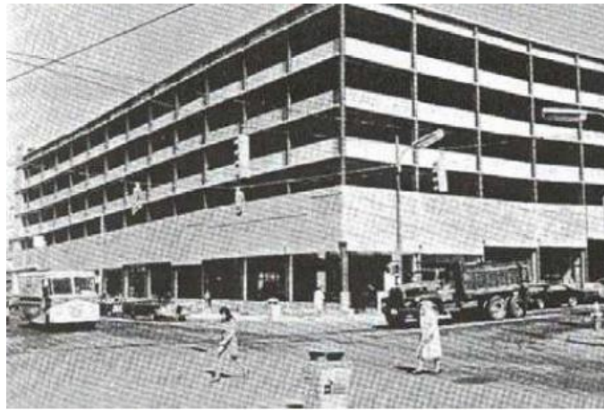
Figure 6 - Open car park in Pennsylvania – Gewain (1973 [20]).
