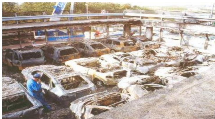
Figure 8 - Fire in car park of Schiphol airport [24].
