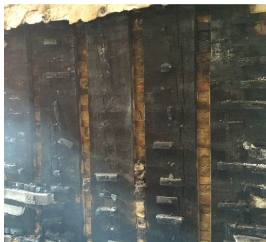
Fig. 9 - Timber structure after the test (th = 10 mm)
