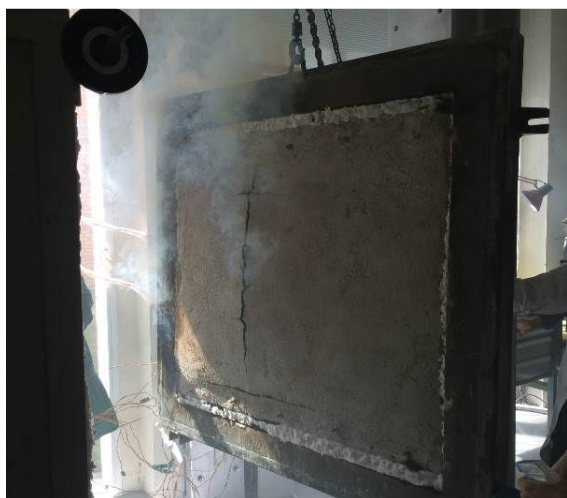
Fig. 8 - Earth-based mortar crack
