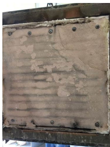
Fig. 10 - Tabique wall panel after opening the furnace door
