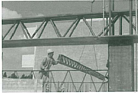
Fig. 1: Original CSTCB with bottom steel plate. [3]
