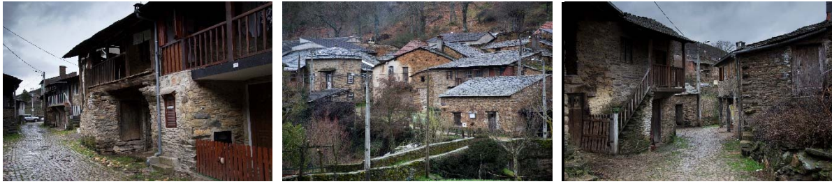
Figure 1: Buildings with schist masonry walls
