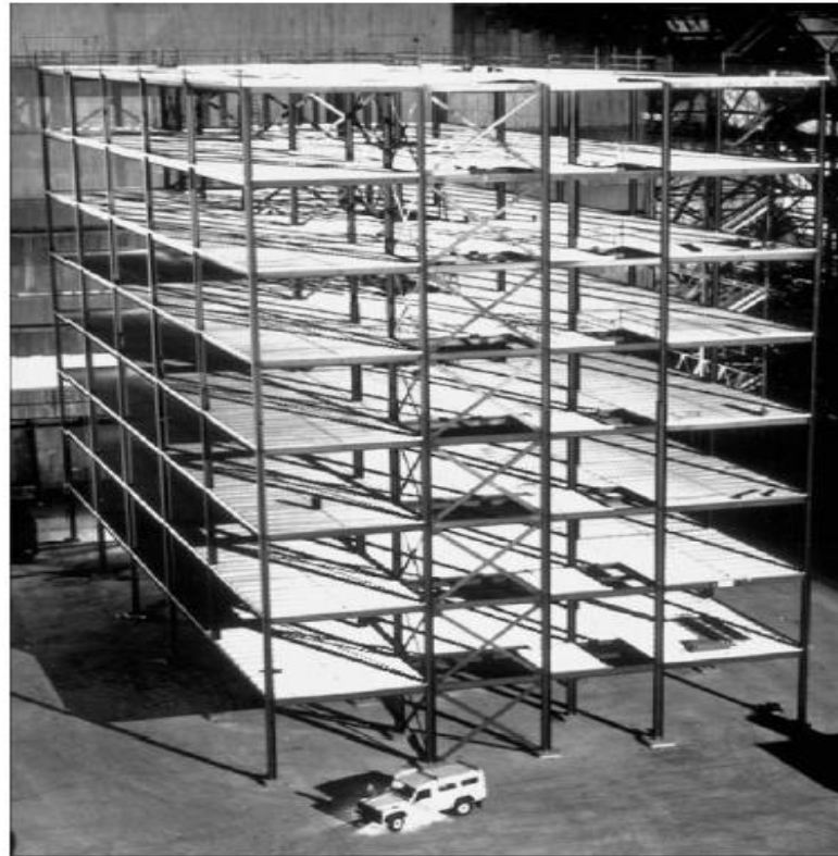
Figure 2.3: Composite steel framed building at BRE Cardington[40].
