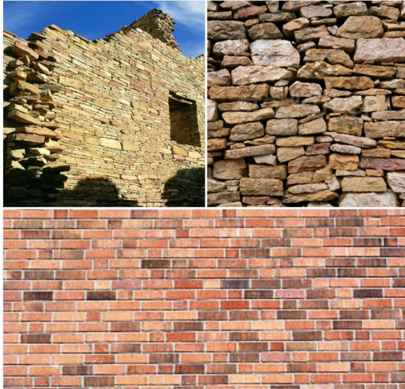
Figure 1-Masonry walls constructed with stones and bricks.
