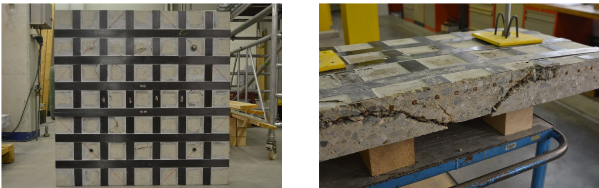
Figure 8 – Cracking pattern and internal shear crack of slab BCG1 after failure
