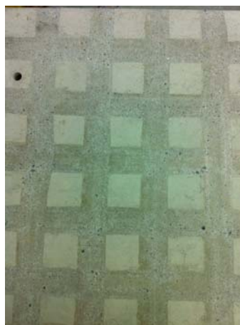
Figure 3 – BCG1 surface prior to CFRP gluing
