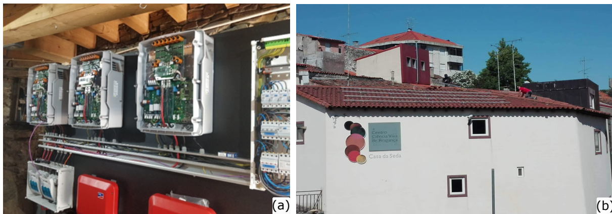
Figure 4.5: Installation process of the (a) microgrid devices and (b) photovoltaic modules.
