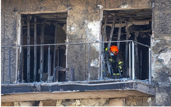
(a) Post fire inspection on Friday.
