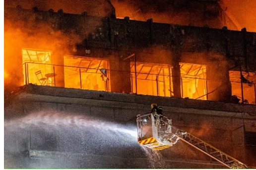
(b) Detail of the facade and interior of the building during the fire.
