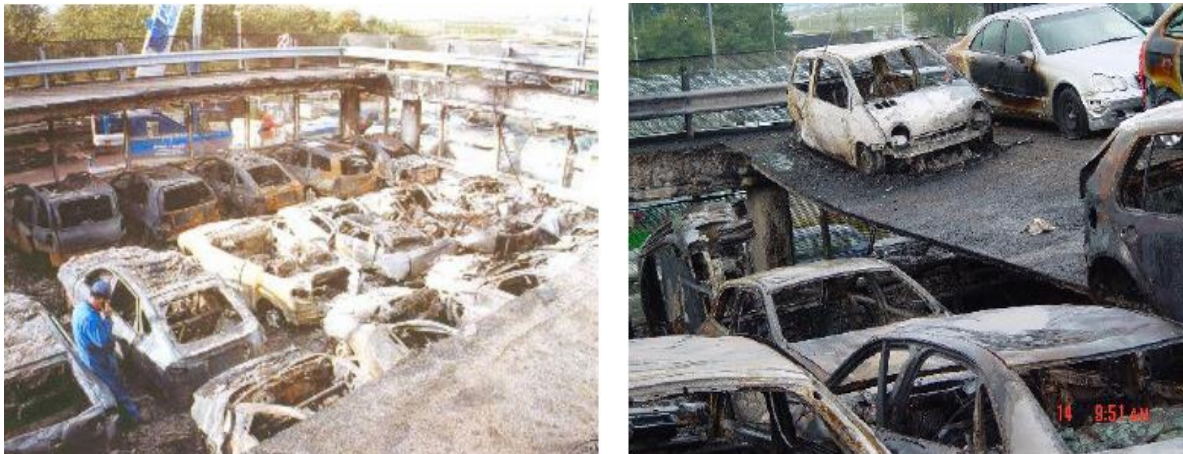
Figure 1: Picture after the fire in the car park near Schiphol airport. [15]
