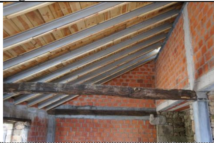
Figure 9. Roof with metal steel beams and wood.
