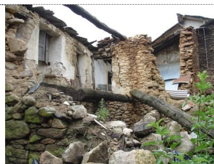
Figure 5. Internal ruin collapse structures.
