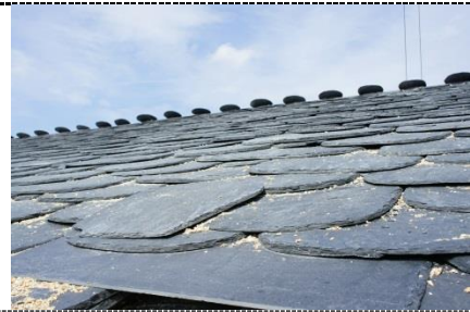
Figure 10. Roof with slate tiles.
