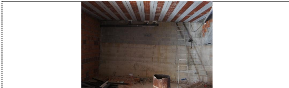
Figure 8. Lateral walls at first floor in concrete.
