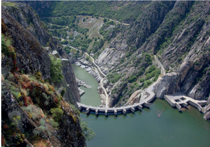
Figure 3: Aldeadávila Dam in the Arribes del Duero (Spain– Portugal). Picture by Pablo Orduna Portús
