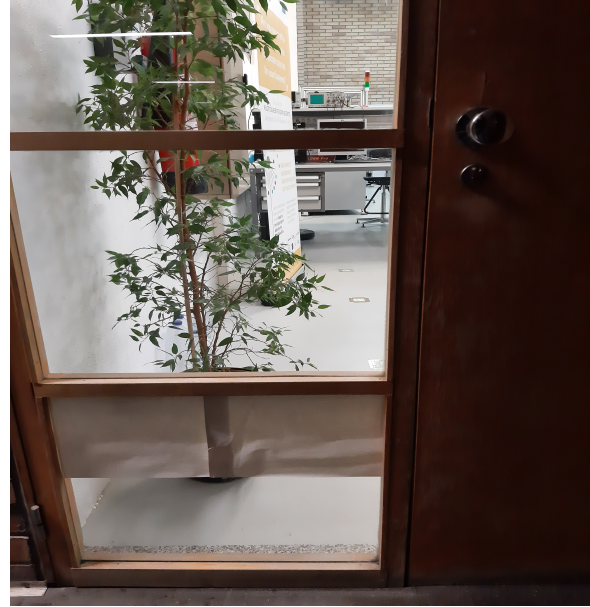
Figure 5.11: Paper band positioned on the access door of one of the laboratories.
