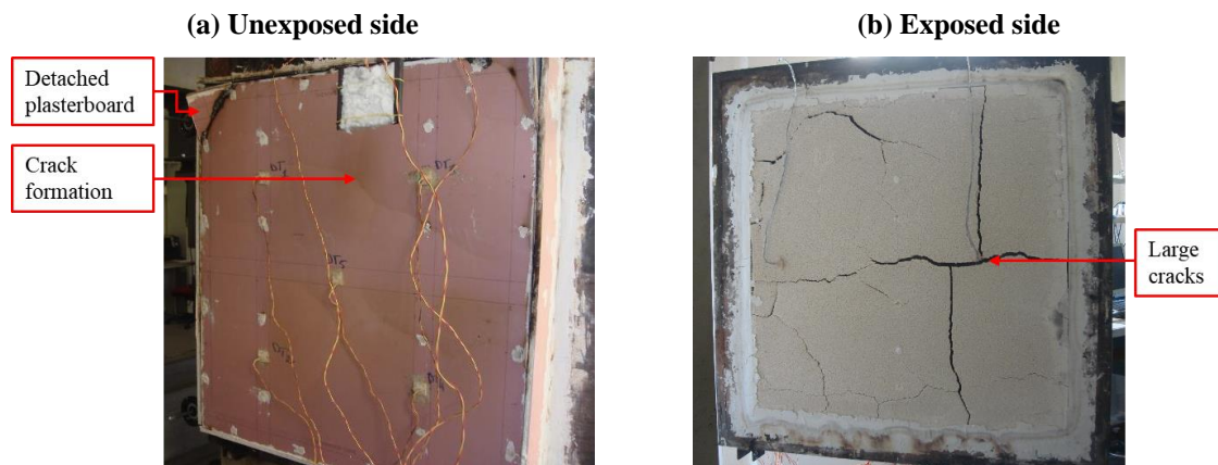
Figure 3.8 – Unexposed and exposed surfaces of Specimen 1 after the fire test.
