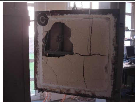
Fall-off of the fire exposed plasterboard due to handling after the test
