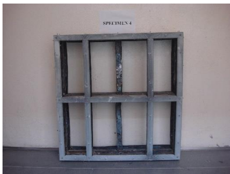
Steel frame condition after the test
