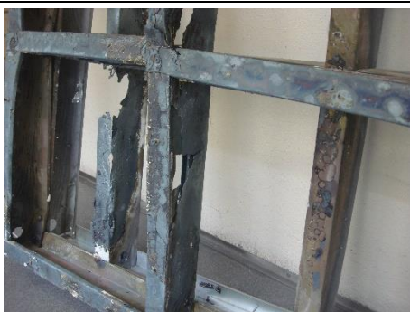
Brittle fracturing behaviour of the steel
