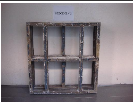
Steel frame condition after the test
