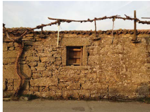
Figure 2. Green wall support system (corbels) on the masonry in Fariza de Sayago , Spain
