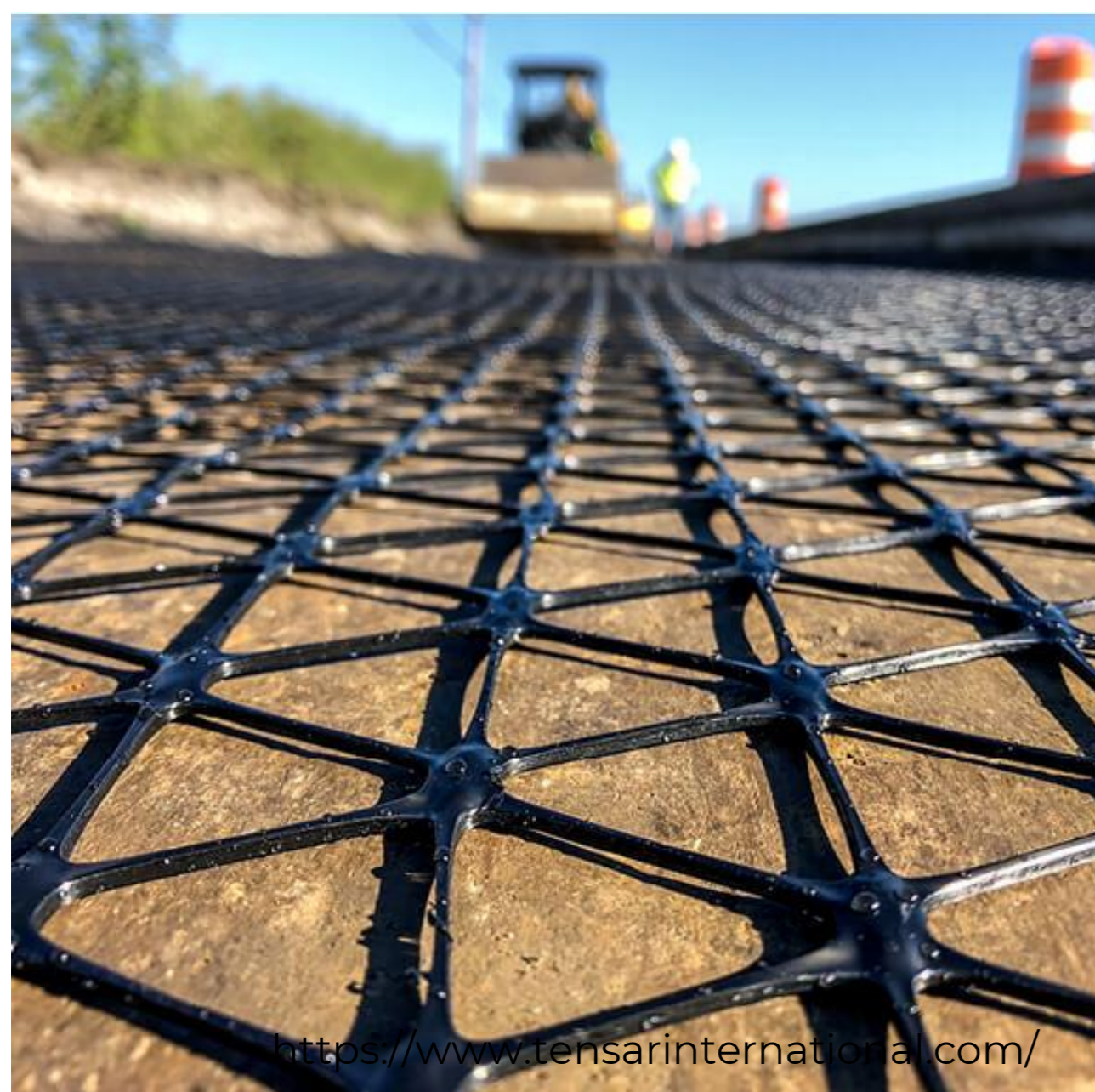
Figure – Geogrid for pavement reinforcement
