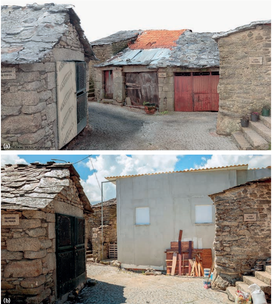
Figure 11. Building intervention record 2: (a) photogrammetry model (2023); (b) current state (2025)
