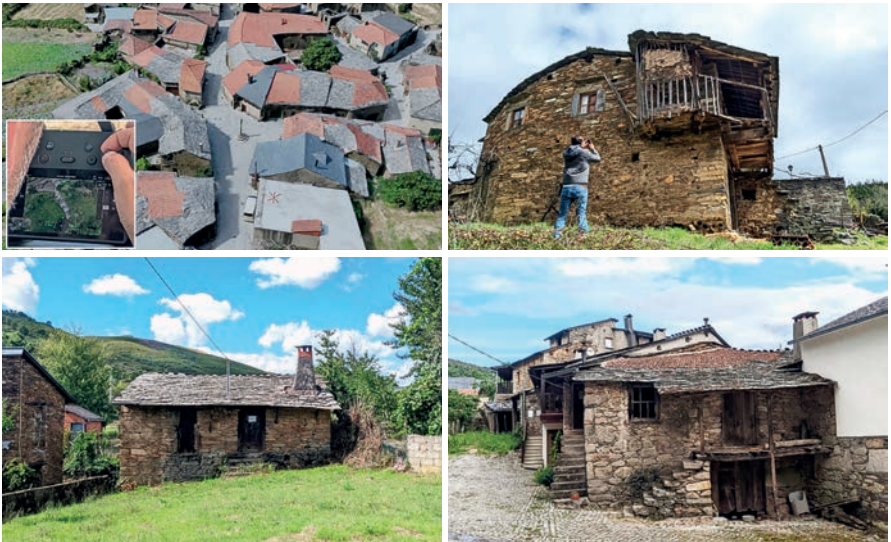
Figure 3. Samples of surveyed vernacular buildings in schist and granite
