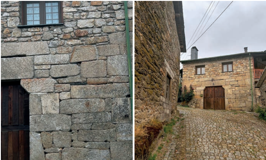
Figure 2. Exterior walls, window frames, staircases, lintels
