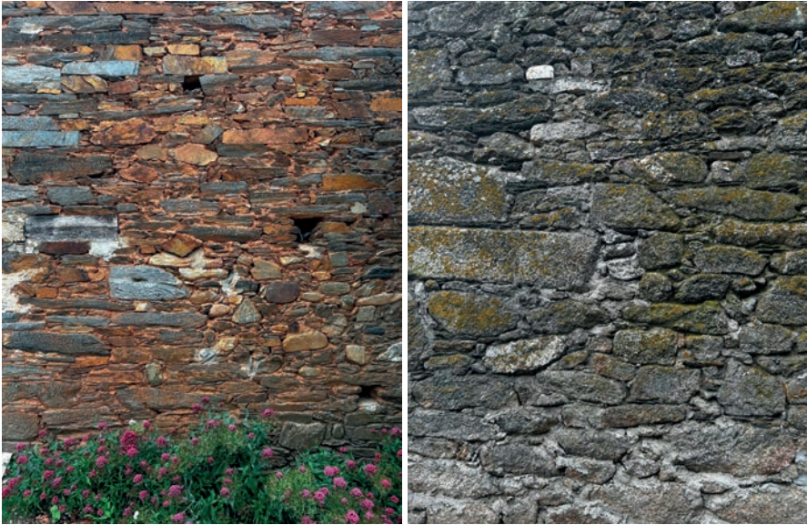
Figure 4. Schist and granite masonry walls details, in França and Montesinho villages
