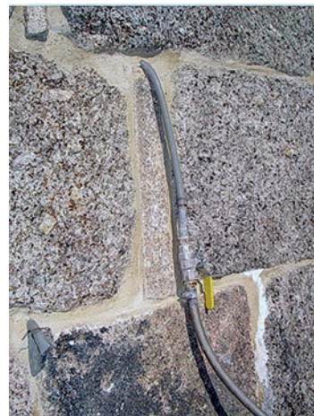
Figure 7. Hand and gravity grouting scheme (Ashurst & Ashurst 1990) and an example of injection
