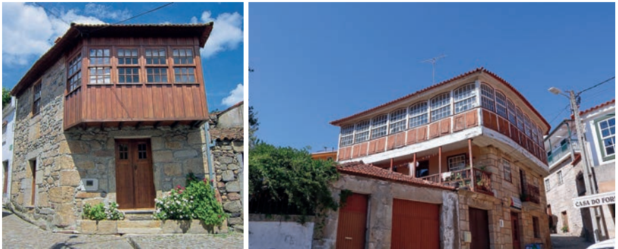
Figure 1. Glazed balconies in Beira Alta – (left) Granja do Tedo, Tabuaço; (right) Salzedas, Tarouca.
