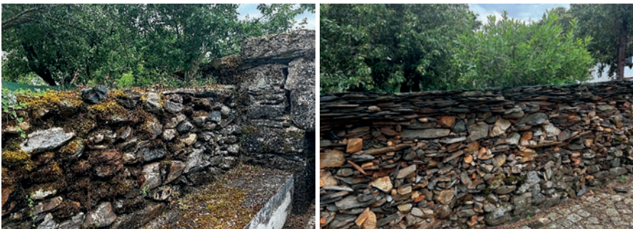
Figure 5. Fencing walls, mills and presses where the dry masonry technique is employed
