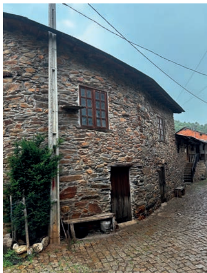
Figure 13. Timber in windows, doors and frames
