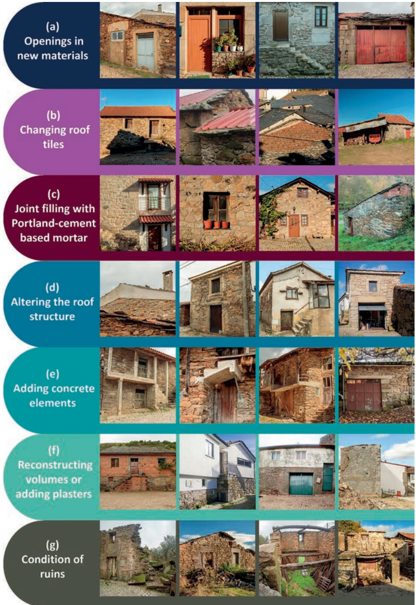
Figure 5. Common physical transformations observed in the vernacular built environment of MNP (Arias-Tapiero et al. 2025)
