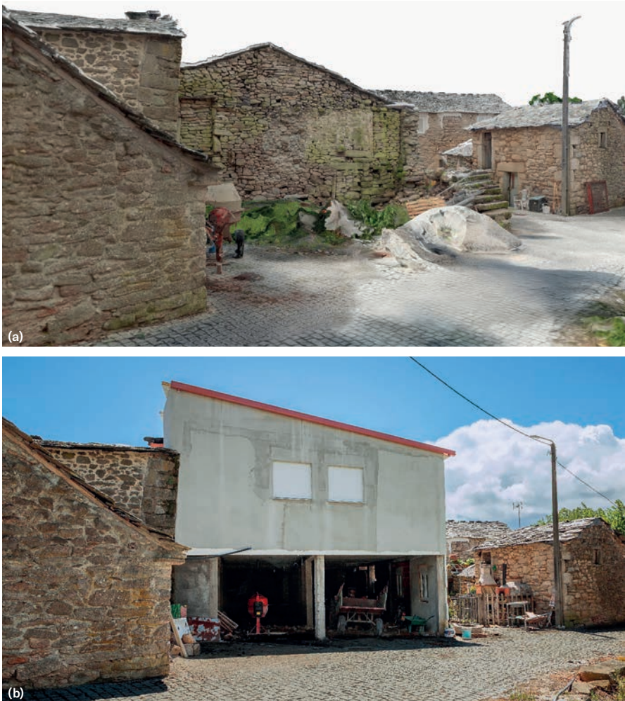
Figure 10. Building intervention record 1: (a) photogrammetry model (2023); (b) current state (2025)
