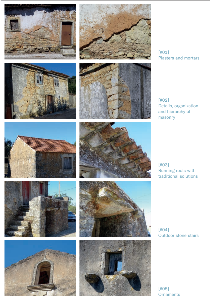
Figure 2. Key elements to the field study of limestone villages (#01 to #05) in pedagogical action 3 (Silva et al. 2021)
