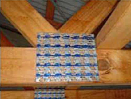
Figure 11: Punched metal plate fasteners, [16].
