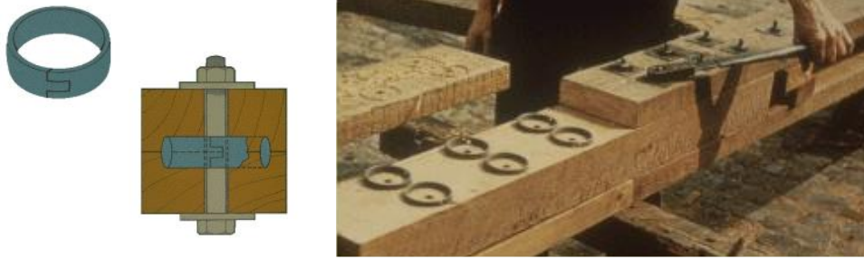
Figure 12: Split-ring connectors with (64- 104 mm) diameter and Bolts (M12 to M20), [16].
