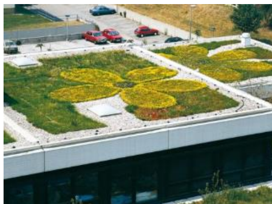
Figura 2.20 – Cobertura extensiva (Green Roof Technology, https://greenrooftechnology.com ).
