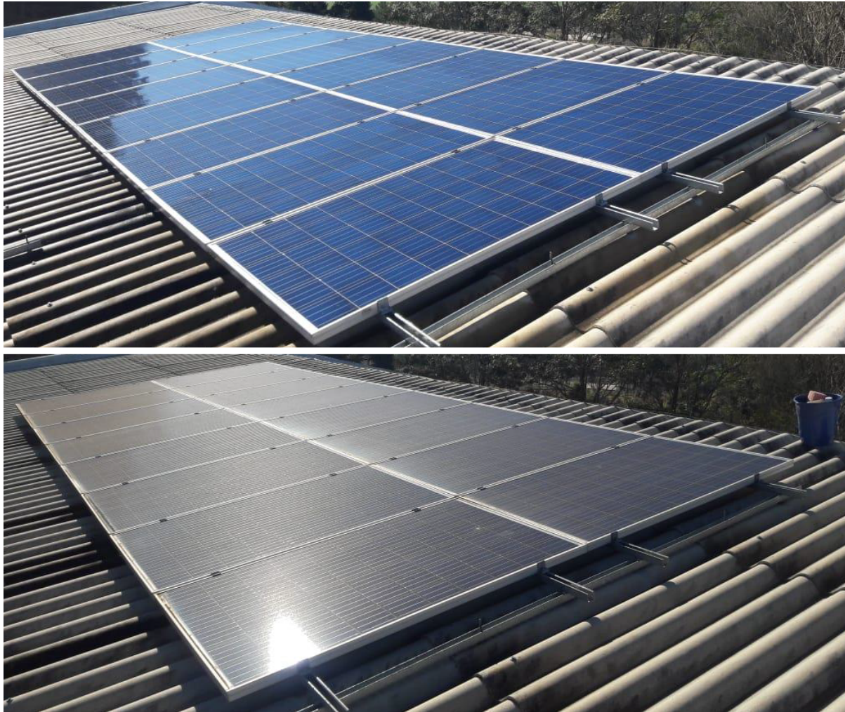
Figure 2.13: Difference Between a Clean and Dirty PV System. [44]
