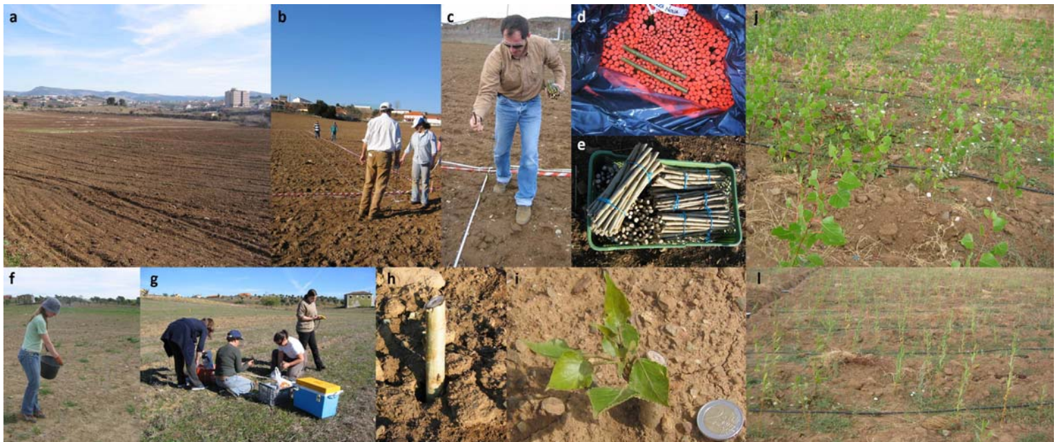
Installation of the experimental SRWC plots in Bragança: a) The area of study before the installation of the crops; b) planting according to the double row system; c) manual planting of cuttings; d) cuttings of Salix ; e) cuttings of Populus ; f) fertilization with phosphorus; g) soil and arthropods samples collection; h) Populus cutting after plantation; i) Populus cutting a month after plantation; j) Populus plot 5 months after plantation; k) Salix plot 5 months after plantation
