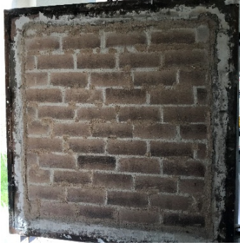
Figure 7: Integrity of the CEBs panel.
