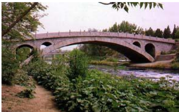
Figura 2.5 - Ponte Zhaozhou, China [Rodrigues, 2011]
