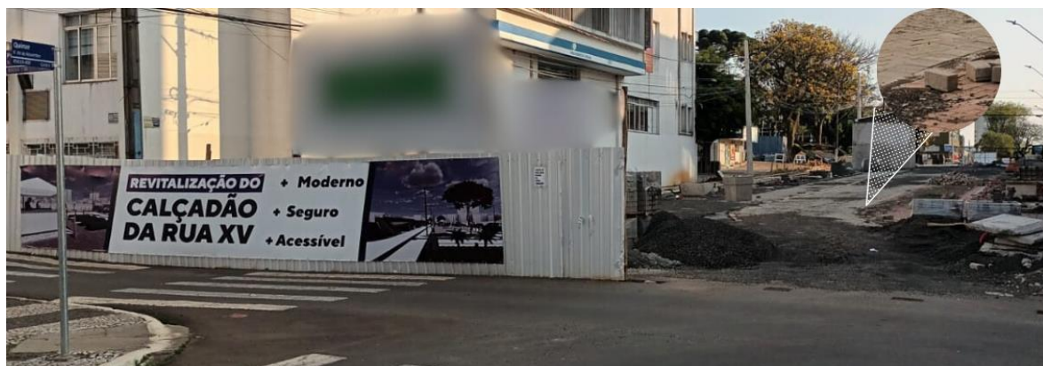
Figure 2 – Execution of the new 15th of November street in paver blocks
