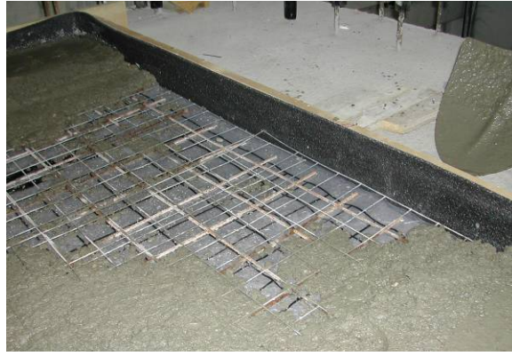
Figure 4.2 - Final concrete layer of floating floor of DIENCA
