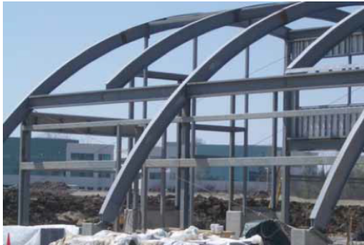
(a) Auto dealership curved roof structure.
