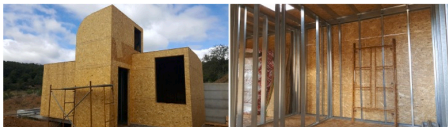
Fig. 1. Example of use of external walls in light steel framing with the use of OSB plates in the region of Coimbra – Portugal (adapted from Ref. [10]).
