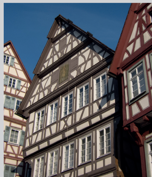
... Traditional timber frame building in the Burgenstraße (Castle Road), southern Germany. (Copyright Thomas Quine, CC-BY, https://archive.is/sdvn7 )
