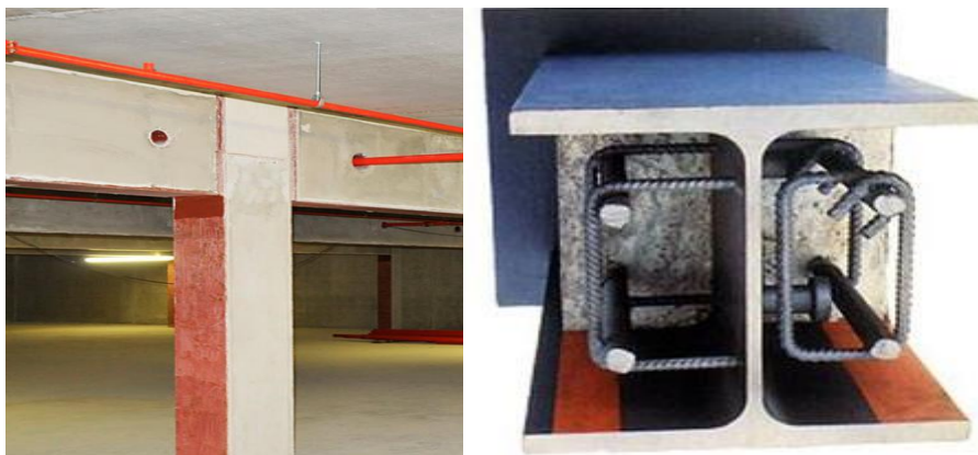
Figure 2: Example of partially encased columns[22]
