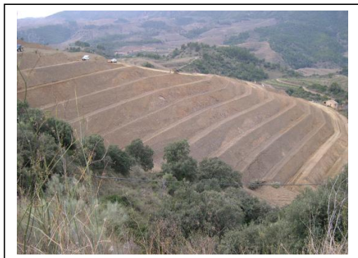
Figure 6: Example of bench terraces constructed at present with heavy machinery in the Priorat region.
