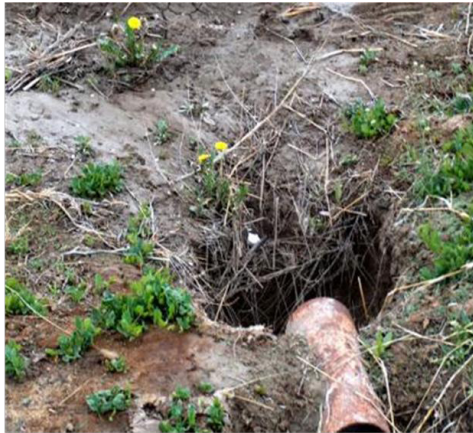
Figure 11: Erosion from simple pipe diversion
