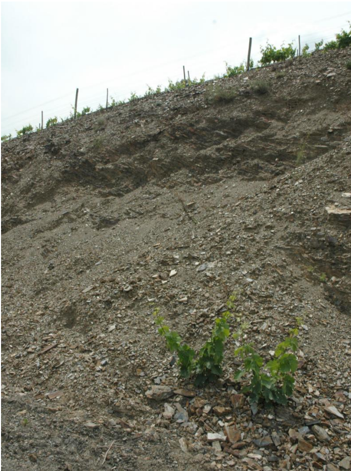
Figure 9: Mass movement produced by the collapse of a border in an area with excessive filling of materials and high slope degree. The foot slope vine row has been buried by the moved materials.
