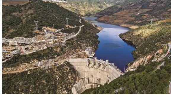
Figure 3. 1: Dam and reservoir (15).
