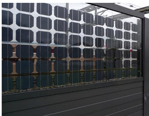
Figura 9: Painel solar BI-PV [8].
