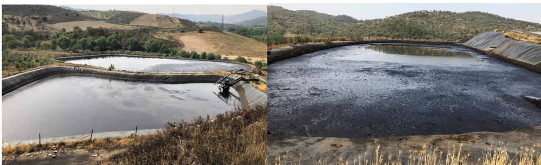
Figure 2: Evaporation ponds of the olive pomace oil extraction wastewater.
