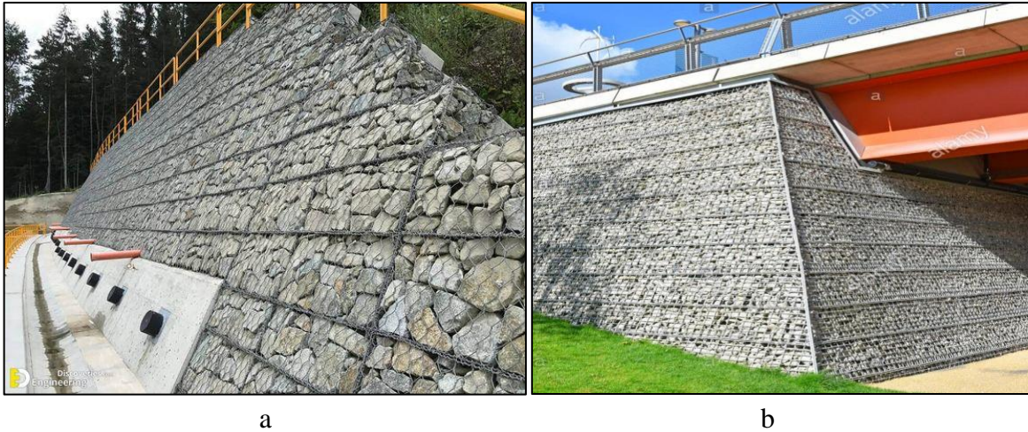
Figure 1.11 Gabions in engineering structures: a – gabion caged basket in bridge abutment; b – gabion retaining wall. [31]
