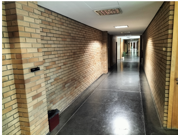
Figure 5.11: Module placed on the corridor wall.
