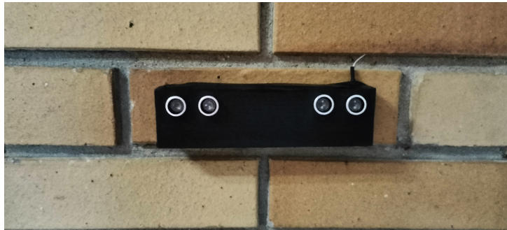
Figure 5.10: Module placed on the wall.
